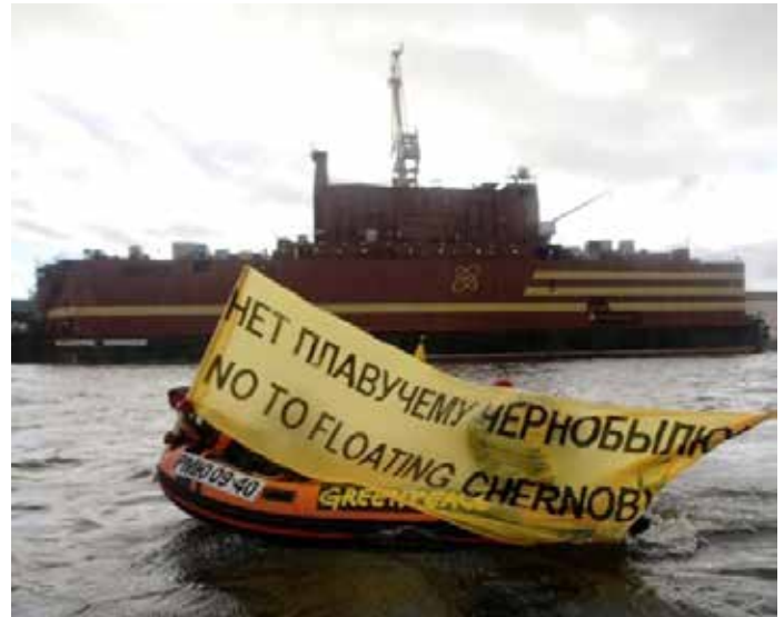
Russia's floating nuclear power plant will be used to power fossil fuel mining operations in the Arctic. Photo: Greenpeace
