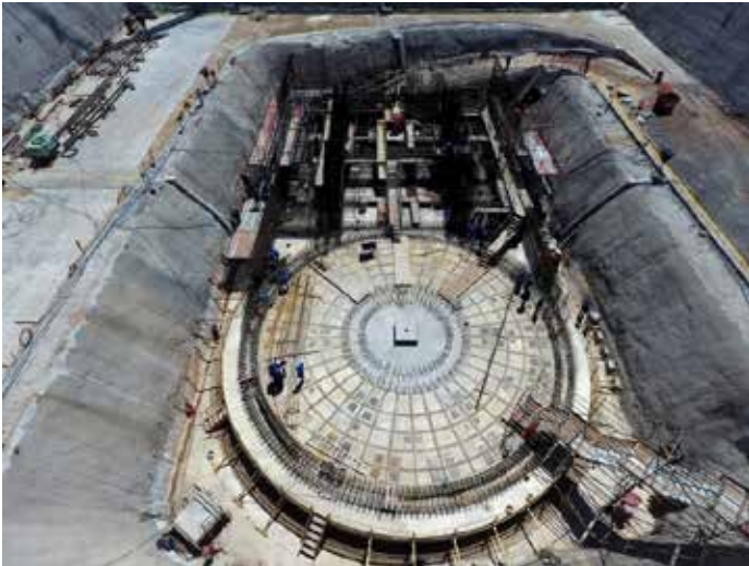
The CAREM SMR under construction in Argentina.
